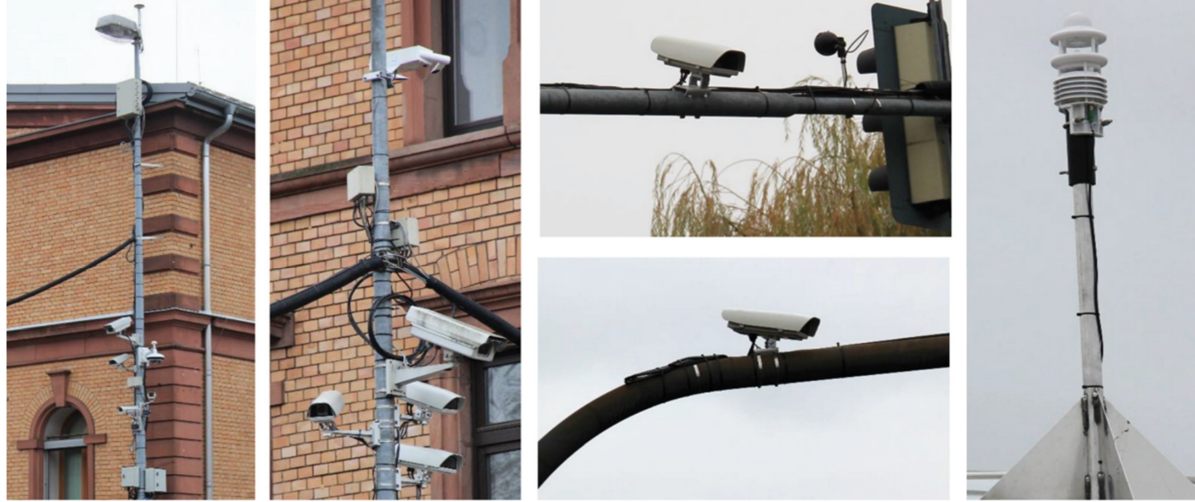
Fig.1: Multiple sensor positions and types at the Aschaffenburg Research Intersection.
